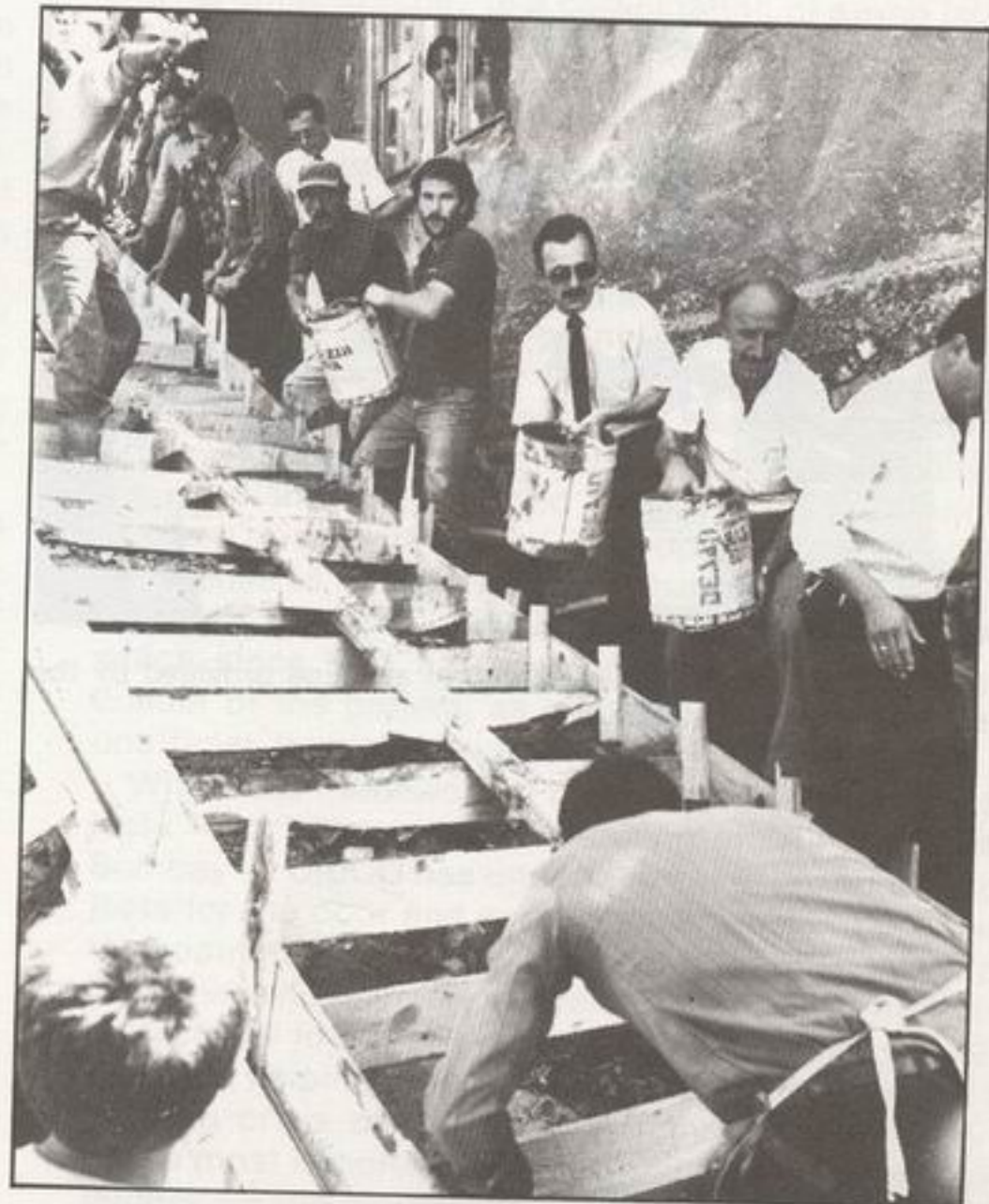
Fig. 4: Pouring concrete for the construction of the first stairway in Zafertepe.
