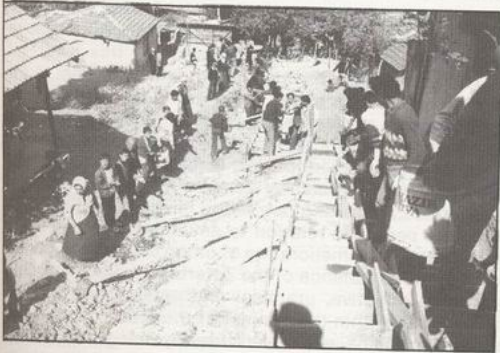
Fig. 2: Zafertepe people working together.
